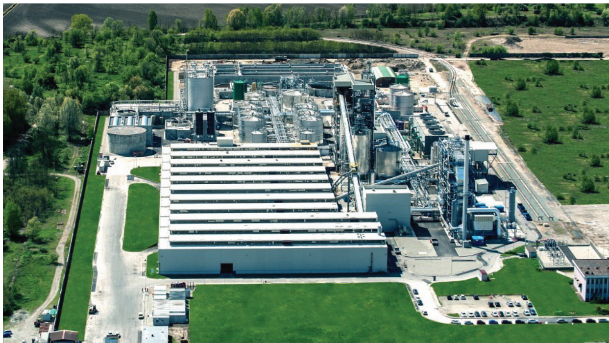
Figure 19 – Biochemtex-IBP – 40,000 ton/y second generation bioethanol plant – Crescentino, It
